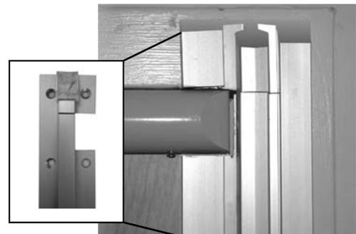
Electrified Power Transfer Hinge
