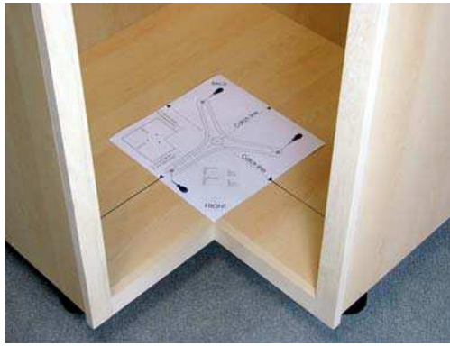
2. Put in the drilling template
