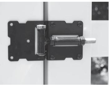
This picture shows the normal placement of the hinge (attached to gate) prior to fastening it to the post. The gap between the gate and post can be adjusted after hinges are fully attached.
