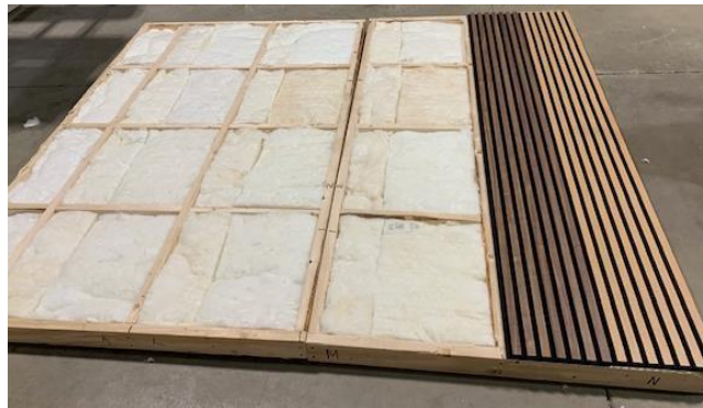
Figure 4 – Panel installed on mineral wool
